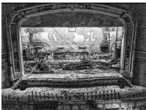
03 - Abandoned and Burned High School Auditorium in Detroit.jpg
